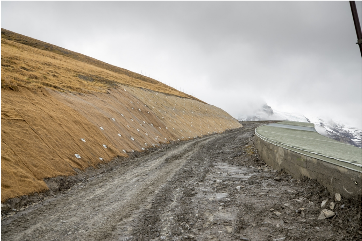
Jungfrau Railway Gallery and blue runway. The embankment is secured with jute nets and anchors. First comes the dung, then the net, which will be covered over in time.
